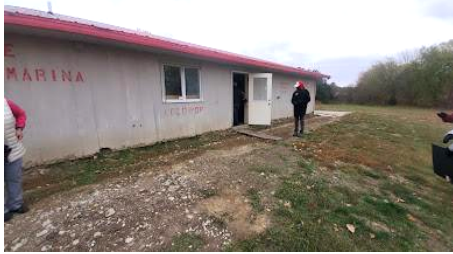
"Year 1" - Old Dilapidated Marina
